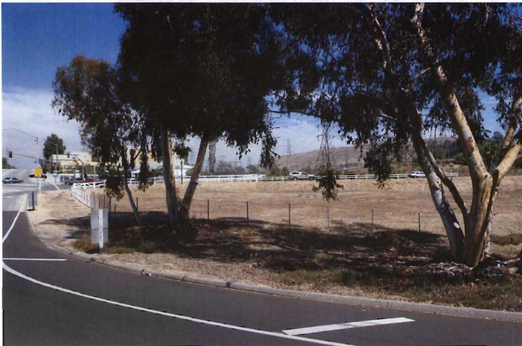
From Freeway Off-ramp looking East Existing
