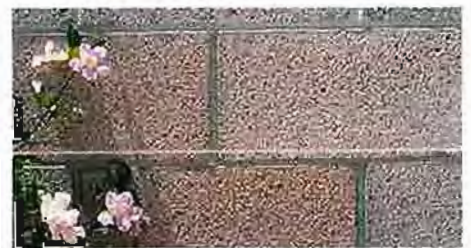
6' High Perimeter Precision Block Wall
