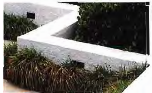
Entry Stucco Wall (36" high) with Stucco Cap
