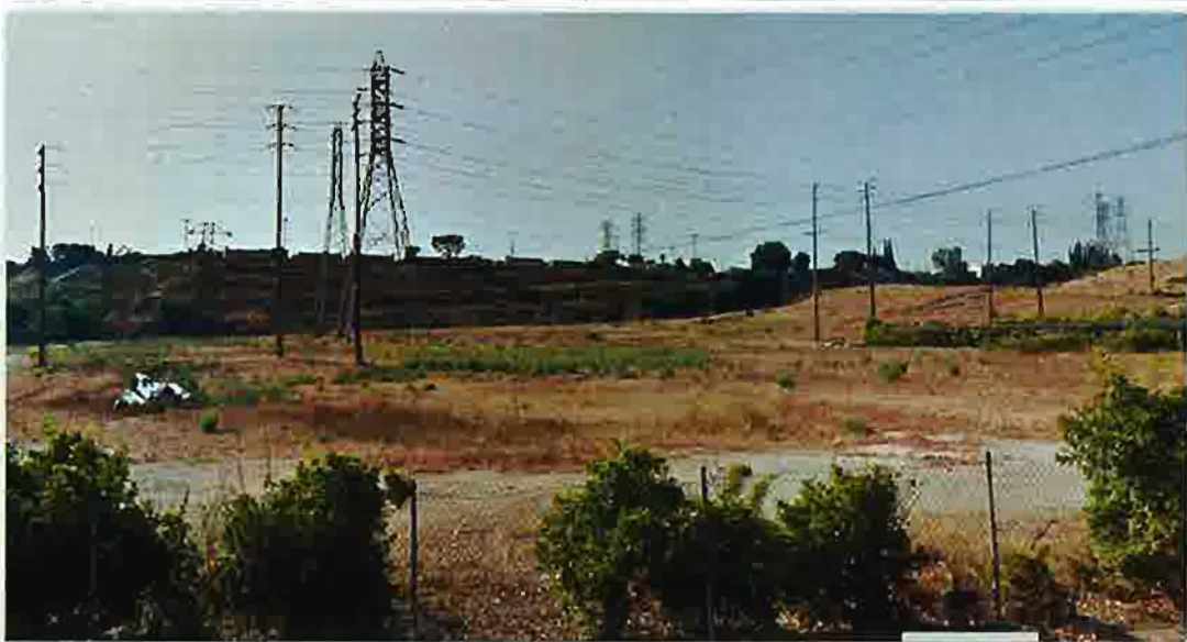
Figure 11. Photo from Potrero Grande Looking North at SCE Transmission Easement West of Site
