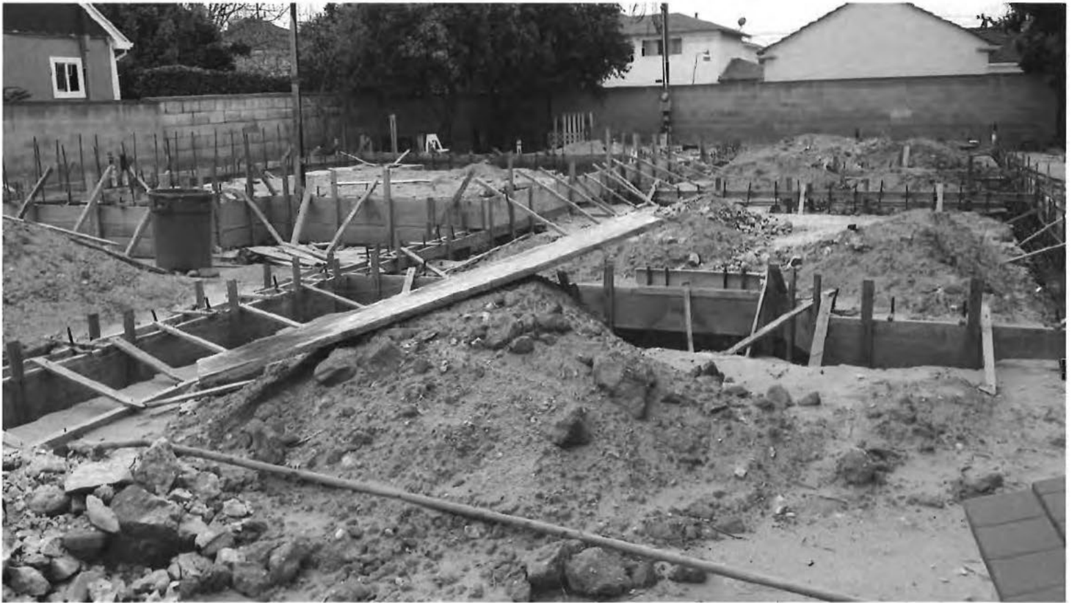
Front View: Current Condition
