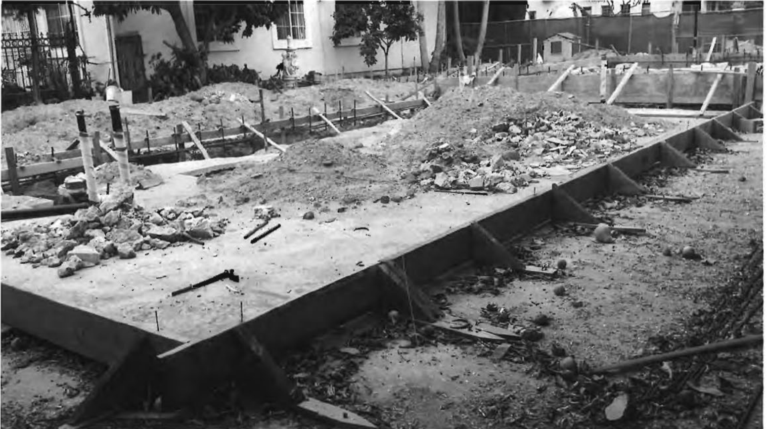
Back Coner View: Current Condition
