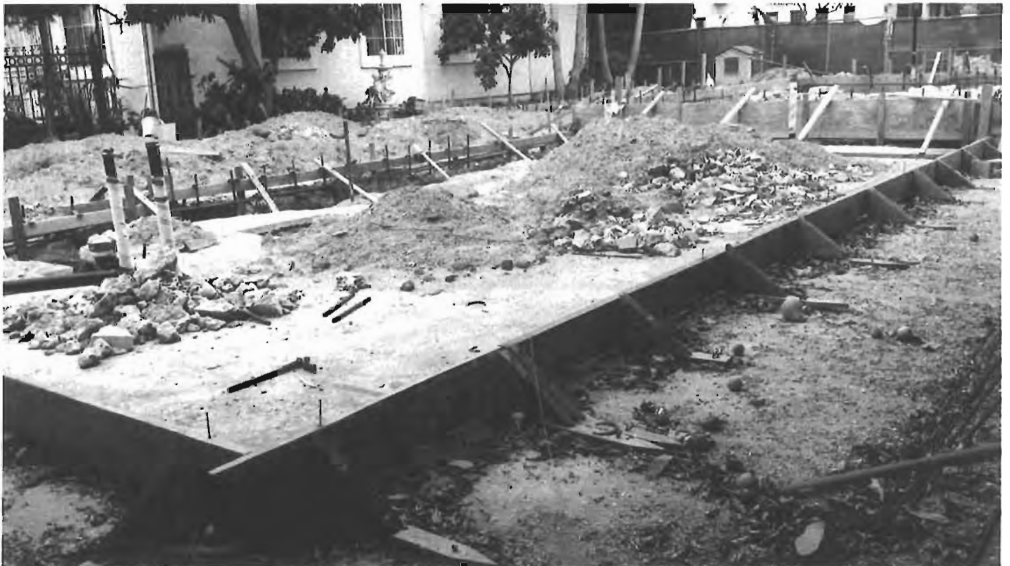
Back Corner View: Current Condition
