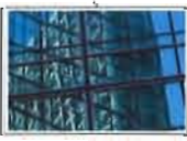
Reflective Spandrel Glass Viracon V903 - Subdued Gray #4 or similar
