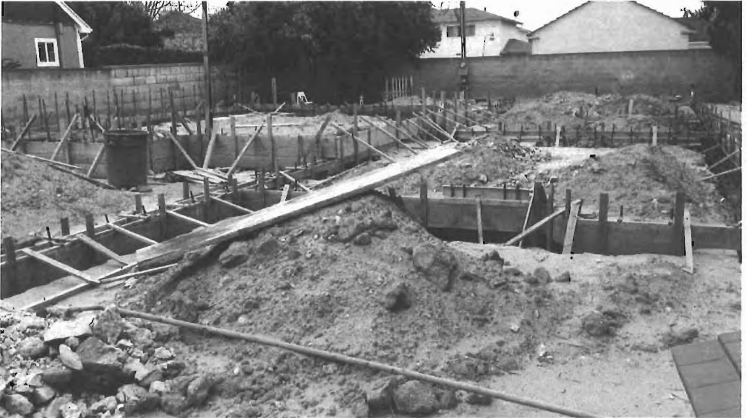
Front View: Current Condition
