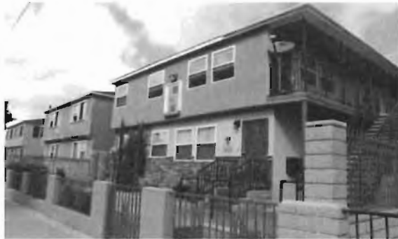
Existing Apartment Buildings:
