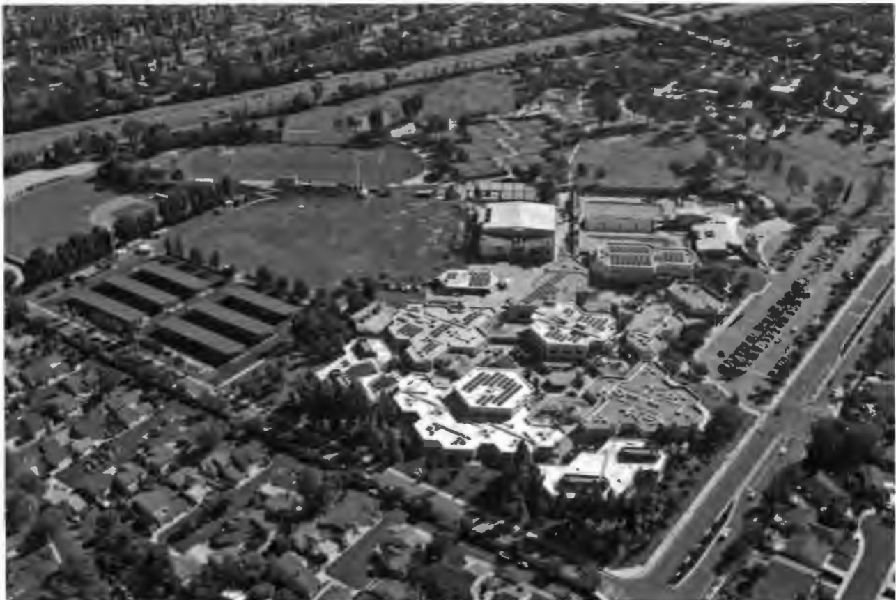
Figure 3: A SunEdison parking canopy and roof installation at the Irvine USD (Irvine High School)
