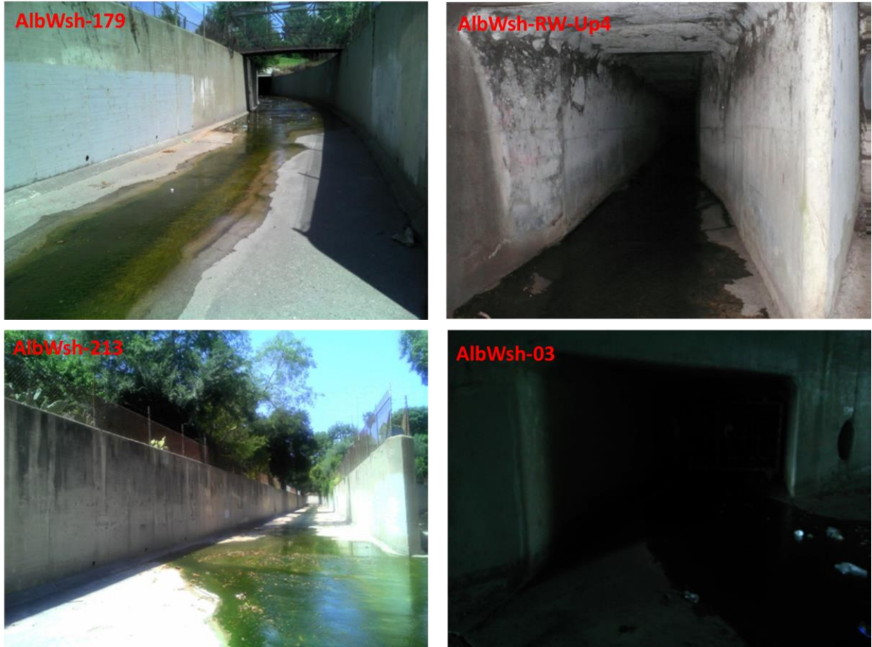
Figure 6.12. Photos of Priority Outfalls in Alhambra Wash (ULAR EWMP Group).
