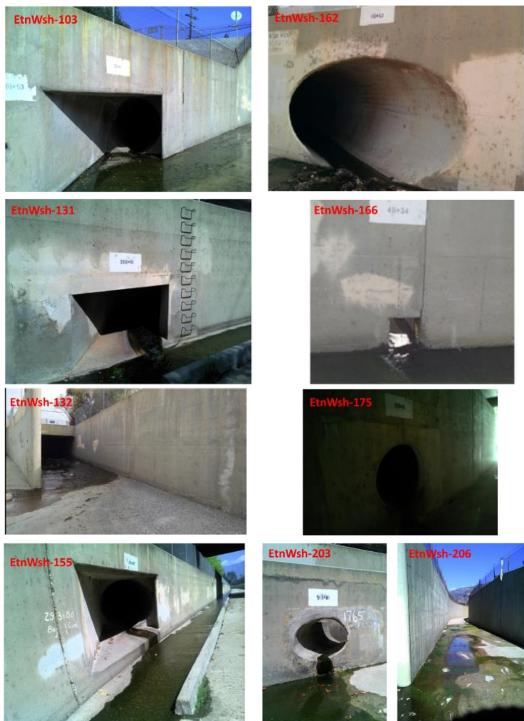
Figure 6.18. Photos of Priority Outfalls in Eaton Wash (ULAR EWMP Group and El Monte).
