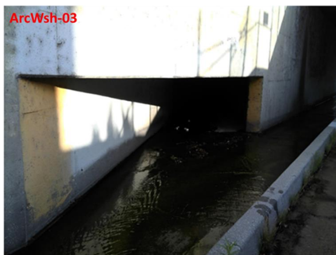
Figure 6.21. Photo of Priority Outfall for Arcadia Wash.
