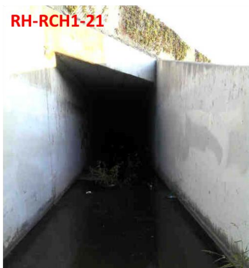
Figure 6.2. Photo of Priority Outfall in Lower Rio Hondo (LA River Upper Reach 2 Group).
