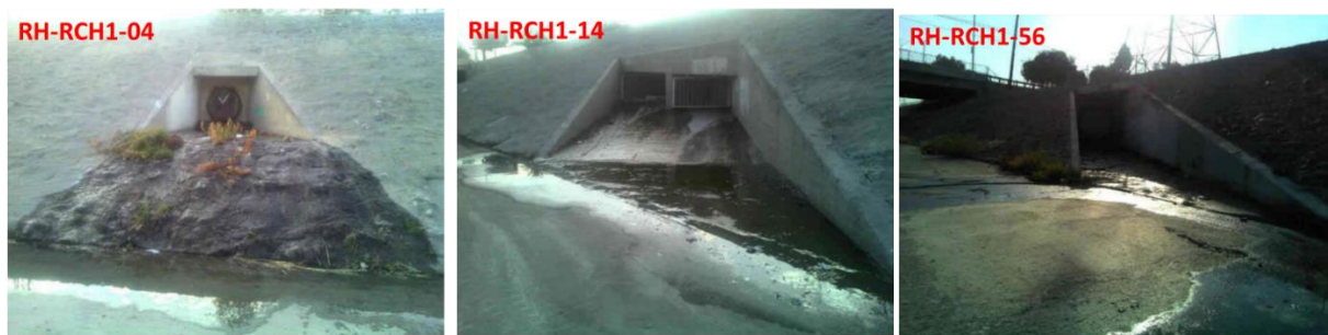
Figure 6.5. Photos of Priority Outfalls in Lower Rio Hondo (LLAR WMP Group).
