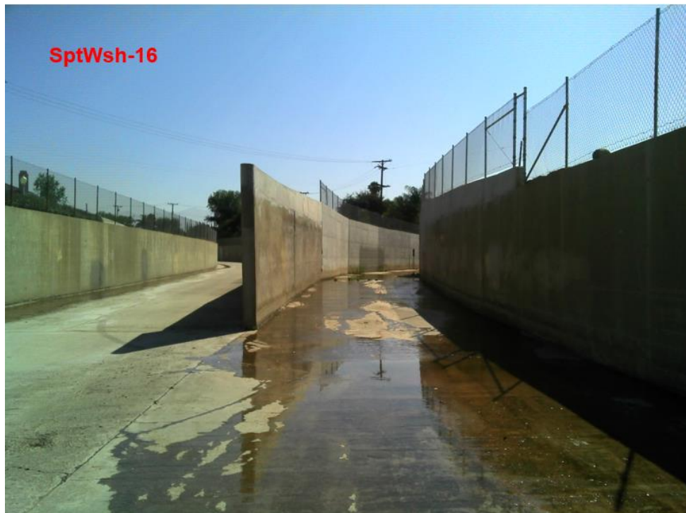
Figure 6.24. Photo of Priority Outfall for Sawpit Wash.
