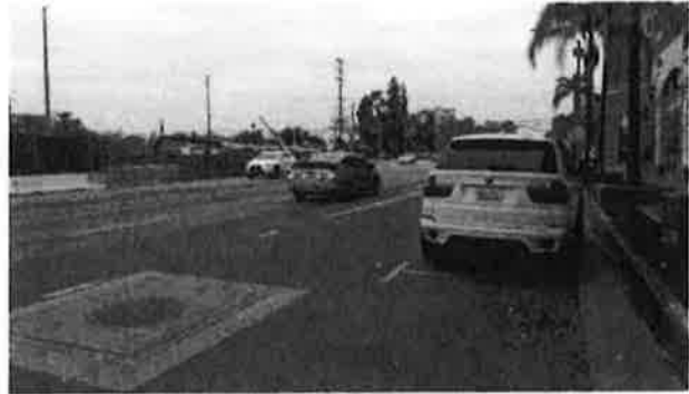
PHOTO 2: SOUTHERN CALIFORNIA EDISON MANHOLE ON ATLANTIC BLVD. NEAR HELLMAN AVE.
