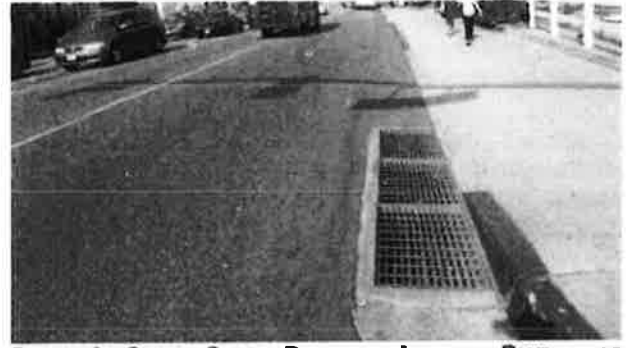
PHOTO 6: GRATE CATCH BASIN ON ATLANTIC BLVD. NEAR GARVEY AVE.
