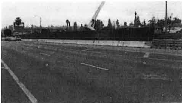
PHOTO 7: NEW DEVELOPMENT CONSTRUCTION LOCATED ON ATLANTIC BLVD., SOUTH OF W. HELLMAN AVE.
