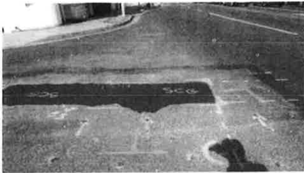
PHOTO 5: RECENT SOUTHERN CALIFORNIA GAS WORK AT THE INTERSECTION OF MABEL AVE. AND ATLANTIC BLVD.
