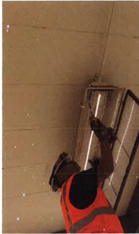
Figure 5 – LED lighting tube being installed
