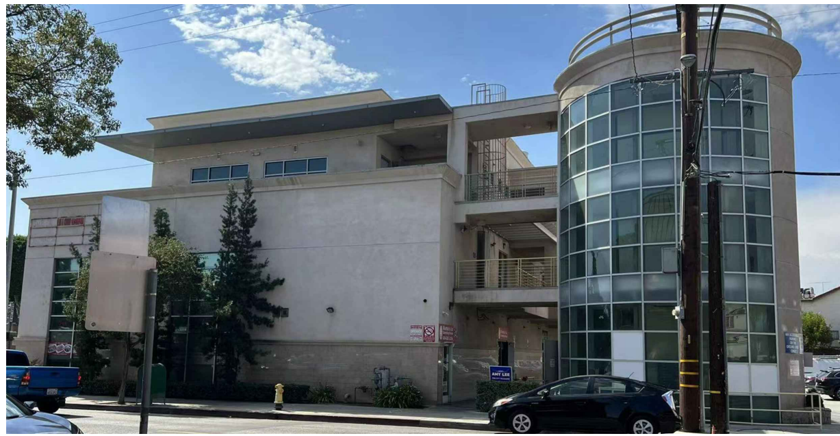
SITE PHOTOGRAPH 1A
